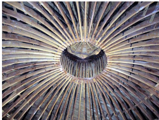
Figure 8. The Building of the Board of Guardians. Full reconstruction of the original (authentic) framework of the internal cupola using whole timber
