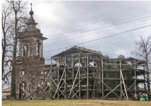
Figure 10. The Cathedral of the Transfiguration of Christ in vil. Snoved. At the time of observation the wooden structures of the cupola had been brought down
