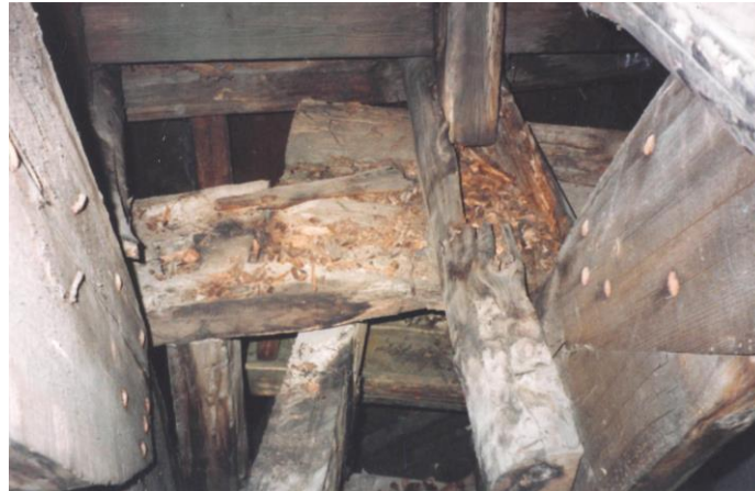
Figure 6. The Building of the Board of Guardians, destruction of the wood
