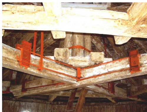
Figure 2. The main house of Ostankino estate. Reinforcement of tightenings of the main arches and elements of the framework by means of steel tension bars with stop channel bars and splice pieces of wood boards
