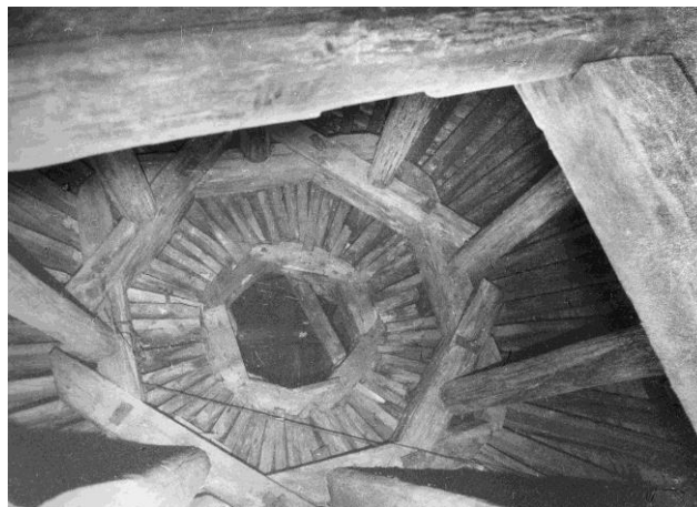
Figure 4. Petrovsky Putevoy Dvorets in Moscow. Separate elements, including the central support - flagstaff base, have rotting and damage from wood fretters
