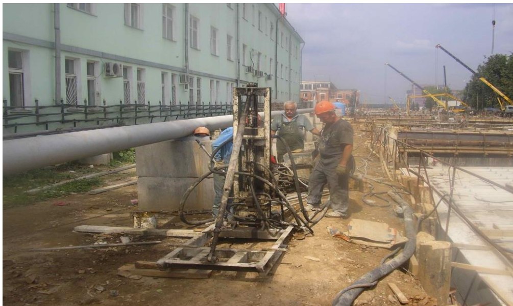
Figure 4. Execution of the cut-off wall between the office building foundation of the flight control tower and the excavation wall of the tunnel
