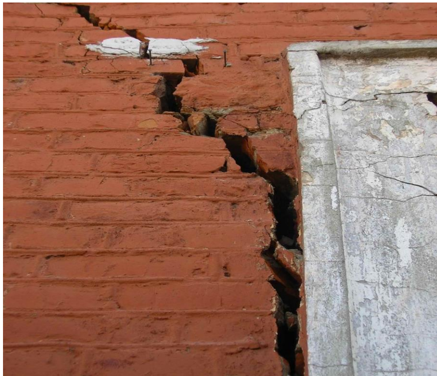
Figure 2. Crack-formation of the aircraft maintenance facility building
