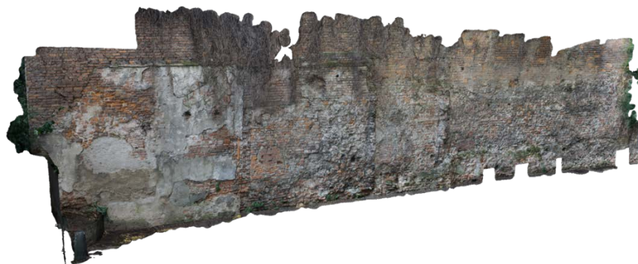
Figure 4. The 3D textured model of the Via Morigi wall, from a photogrammetric survey realized by images captured with a Sony NEX 6 camera coupled with a 24mm F 1.8 Zeiss lens.
