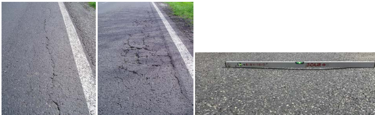
Figure 2. Fatigue cracking and rutting after 3-4 years of open road into service.
