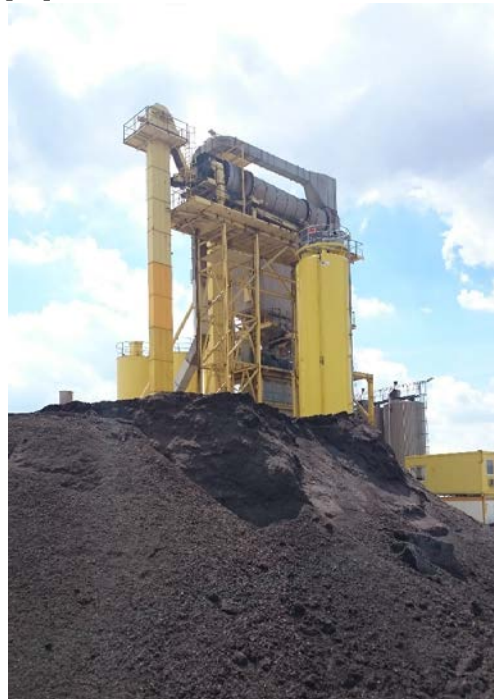
Figure 3. Asphalt plant with RAP drum on the top and view of RAP pile.
