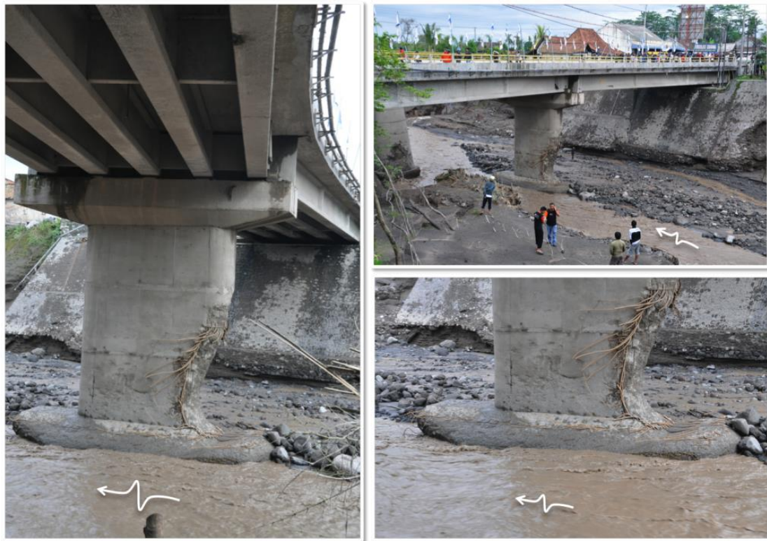
Figure 2. Bridge pier damages on Pabelan River, Pabelan, Jawa Tengah [5]
