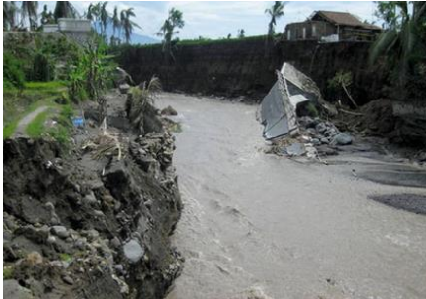
Figure 3. Collapsed bridge due to the destructive of lahar flow [6]
