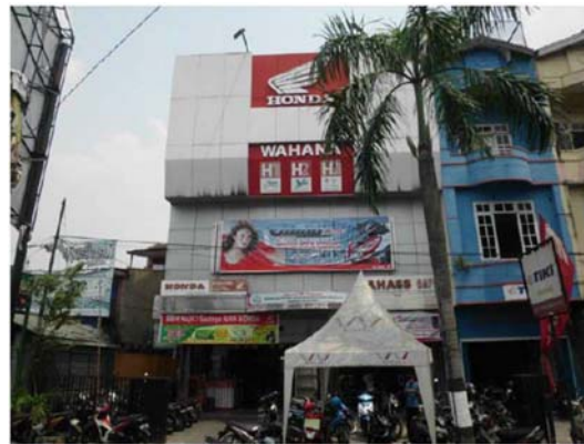
Figure 1. Front View of Wari Medan Building
