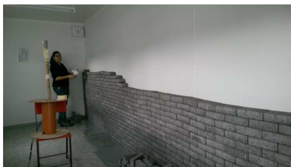
Figure 2. Construction of the concrete accumulation wall
