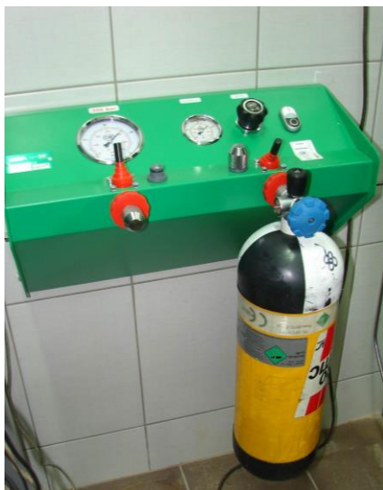
Figure 7. Rapid charge control panel from the air bank
