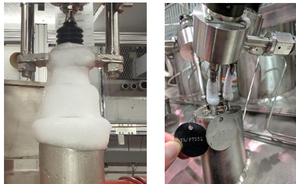
Figure 7. a. Ice formation on the cryomodule JT valve. b. distribution box instrument line.
