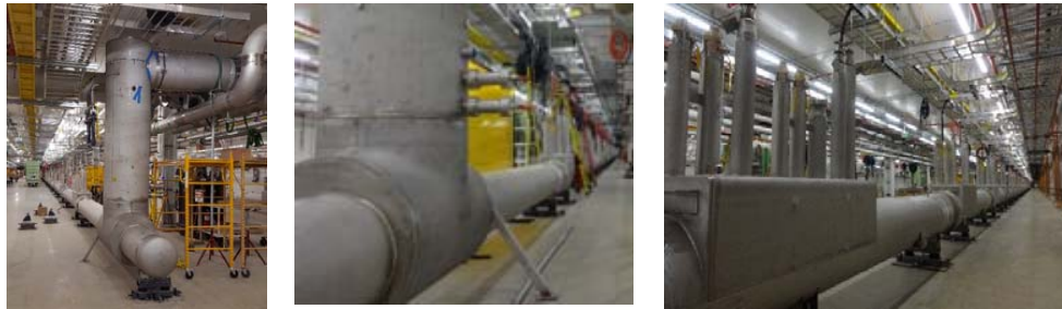
Figure 6. Tunnel cryogenic distribution system installation
