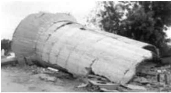
(a) Collapsed circular shaft
