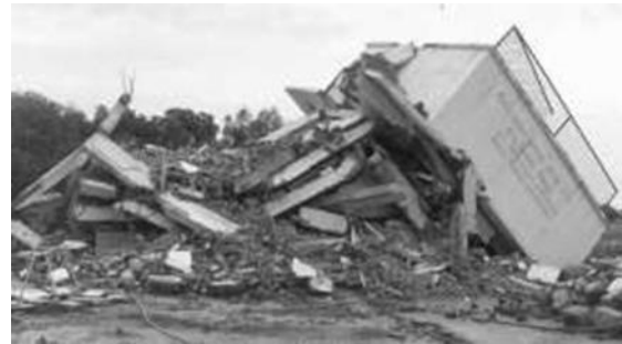
(b) Collapsed weak frame staging
