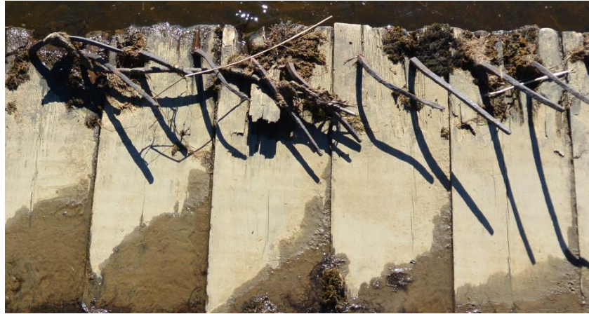
Figure 2. Nails from overturned deck planks. Signs of deformation caused by bending and torque are visible
