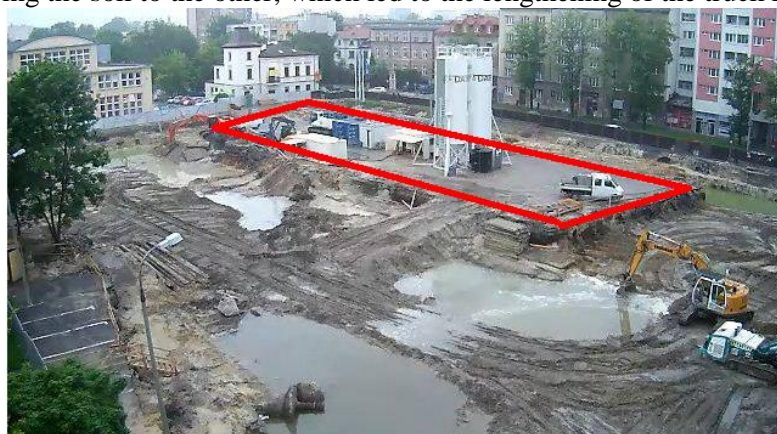
Figure 5. Construction site area with a marked working platform for the machines and for storage of the construction materials (own sources).
