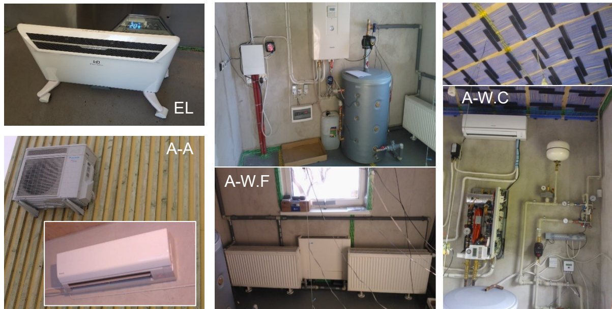
Figure 2. Different heating systems used for heating and cooling: EL – electric heater, A-A – air-air heat pump (used also for cooling), A-W.F – air-water heat pump with convectors, A-W.C – air-water heat pump with capillary mats placed on the ceiling.
