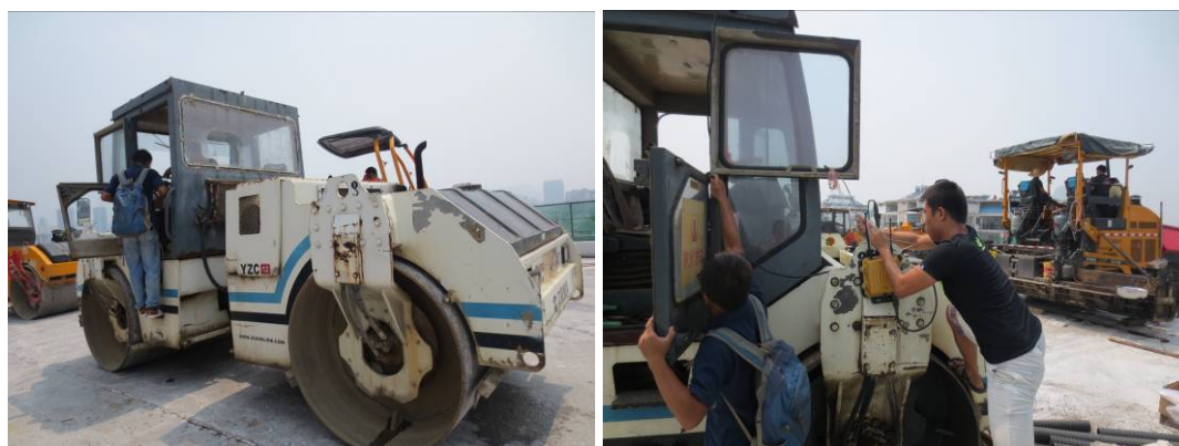
Figure 3. Install the Intelligent Compaction System
