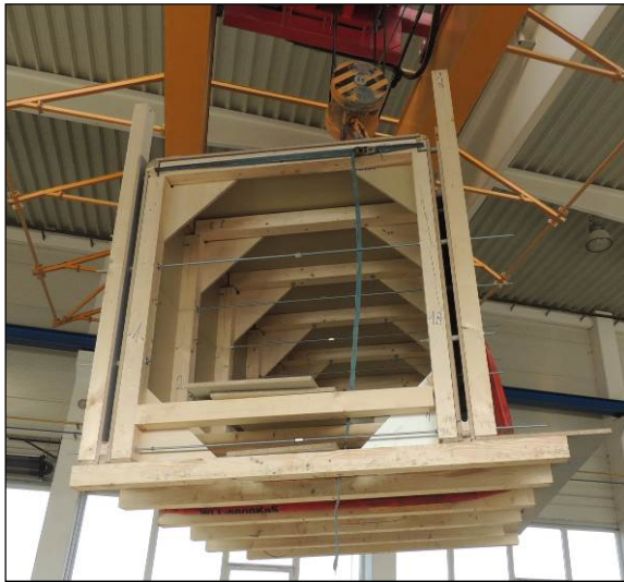
Figure 8. Transport of the 1/4 of the formwork
