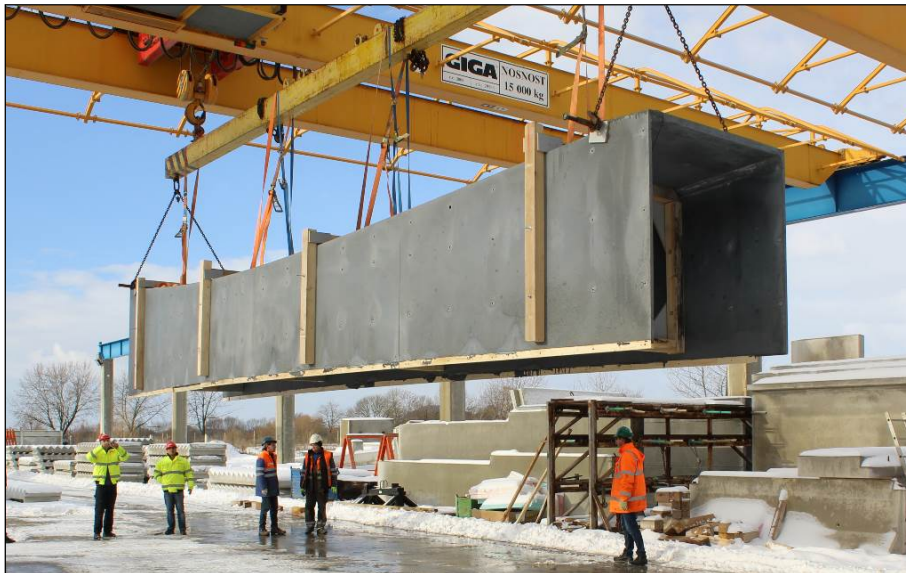
Figure 12. Transport of final 1:1 mock-up of the footbridge in upside-down position
