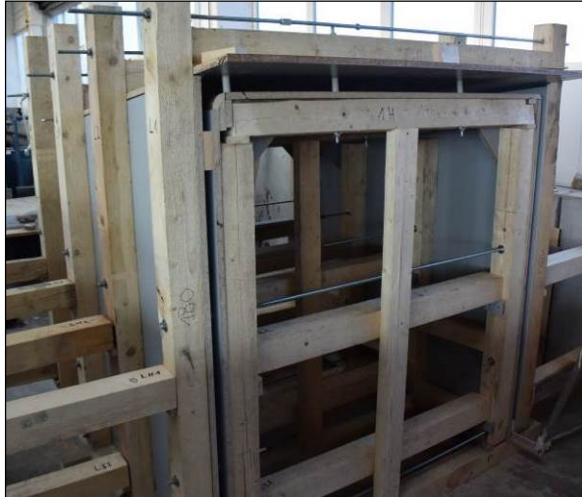
Figure 2. Formwork of the preliminary mock-up
