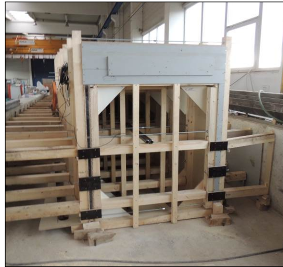
Figure 9. Formwork prepared for the casting
