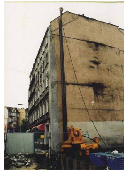
Figure 2. Press-in method
