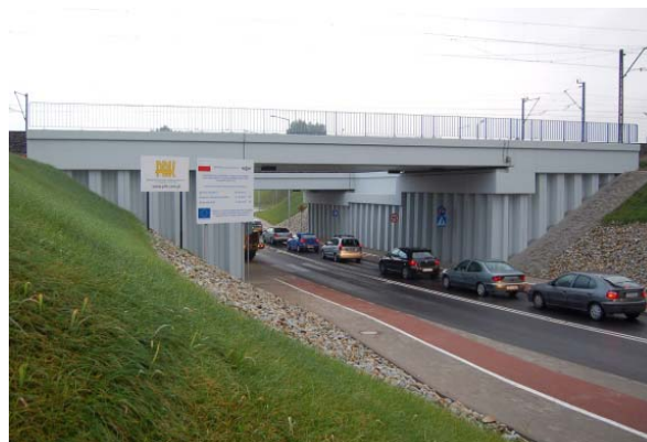
Figure 5. Sheet piles as foundation elements – overbridge in Swarzędz
