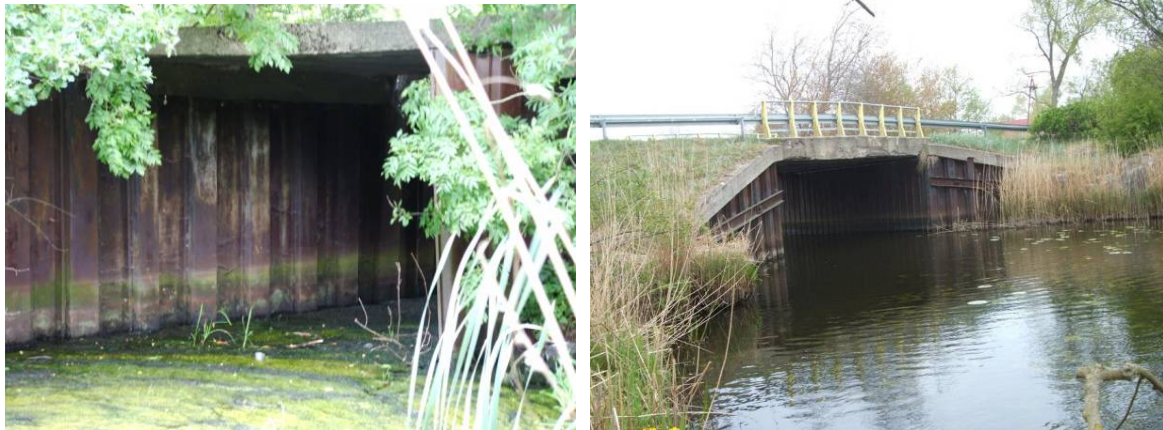
Figure 6. Steel sheet piles in foundation of a bridge in Poland (beginning of XX century structure)
