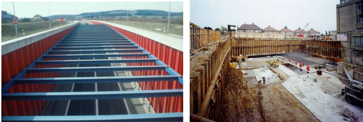
Figure 8. Steel walls with single strut (final wall of tunnel) and anchored (excavation shoring)
