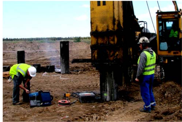
Figure 6. Dynamic load testing
