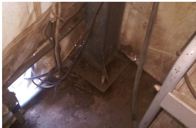
Figure 4. Base plate of a column, with anchoring bolts
