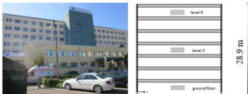
Figure 2. Hospital-type building Nicolae Obalu, Iasi. A vertical scheme for sensors setting
