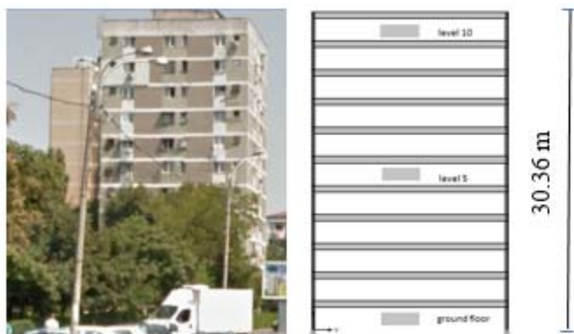
Figure 3. Block of flats-type building, Balta Alba Bucuresti. A vertical scheme for sensors setting
