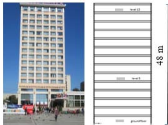
Figure 1. Hotel-type building, Iasi. Vertical layout of sensors.
