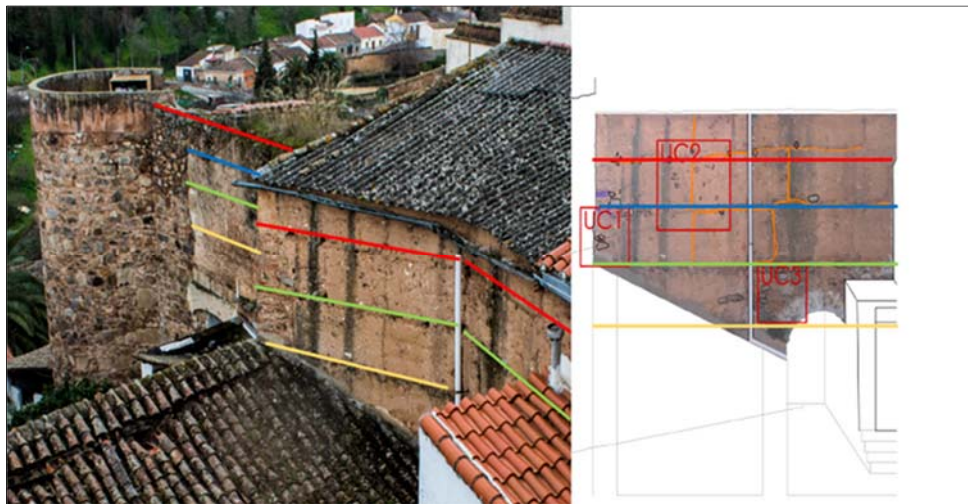
Figure 4. Continuity of the formworks between the original Almohad Wall and the fragment under study.
