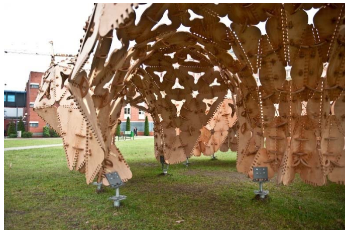
Figure 6. Pavillon was made of plywood panels [38]
