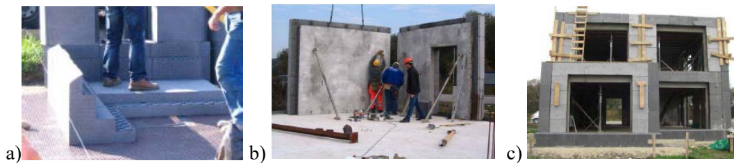
Figure 5. Insulated precast concrete panels EcoB: a) corner elements of EcoB, b) load-bearing panel of external wall, c) EcoB system framework, [14].
