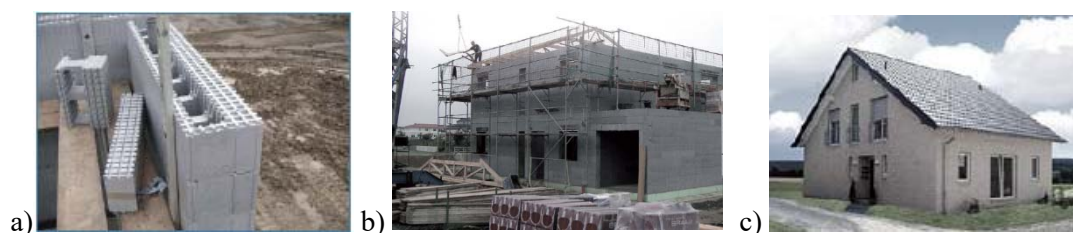
Figure 4. Insulated concrete formwork of Varianthaus system: a) load-bearing reinforced external wall, b) Varianthaus system framework, c) house built by system Varianthaus, [13]
