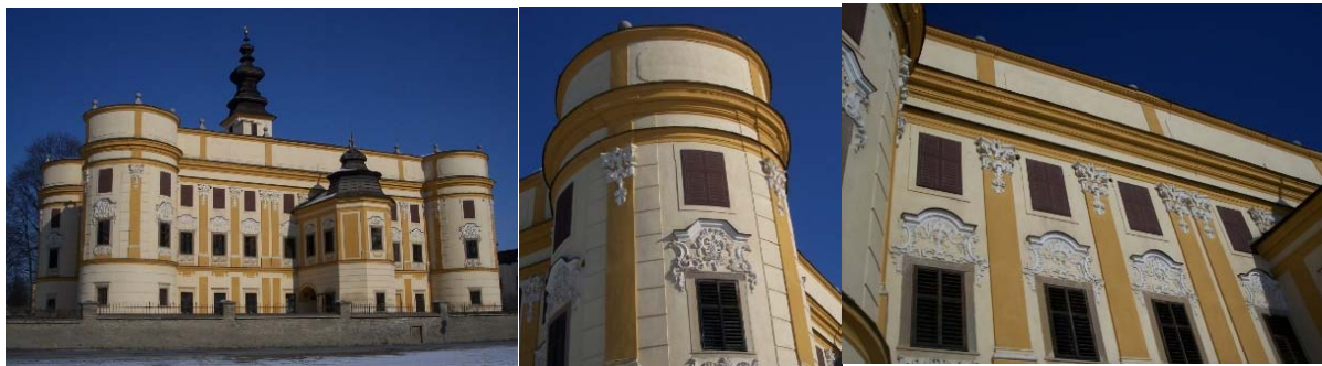
Figure 13 (left). Slovakia, Markuszowce. A Renaissance palace from 1643. All the second-floor windows are the false ones with non-openable shutters. Figures 14, 15. Markuszowce. The first floor windows have openable shutters and the false windows on the second floor have non-openable shutters.
