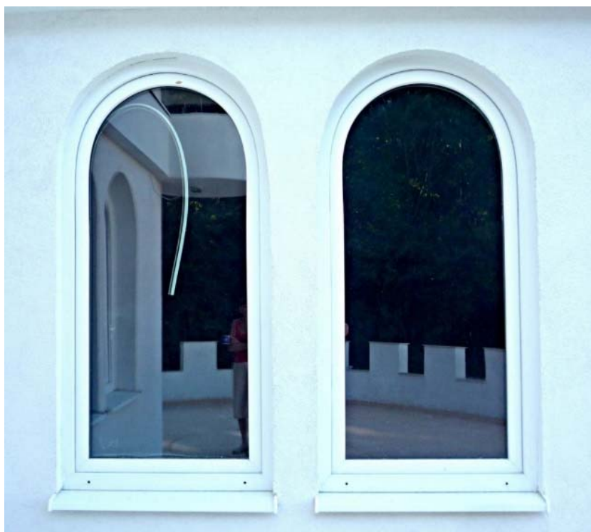
Figure 25. The “Little Castle in Dębogórze” (Zameczek w Dębogórze), two false windows. The loosened window seal resulting from high temperature in the left window.
