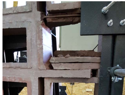
Figure 14. Detail of the destroyed panel
