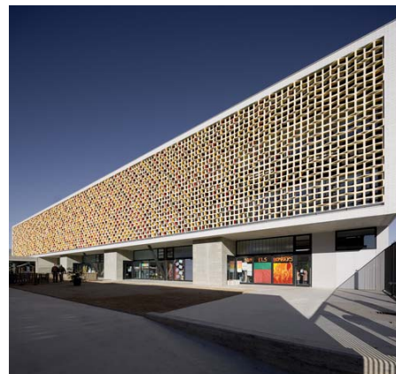
Figure 2. Primary school, Barcelona [4]
