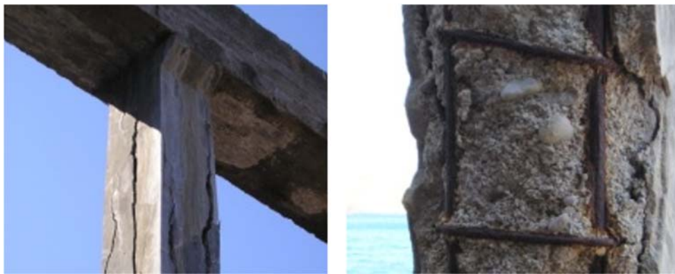
Figure 1. Sample damage to reinforced concrete engineering structures caused by external factors [7]
