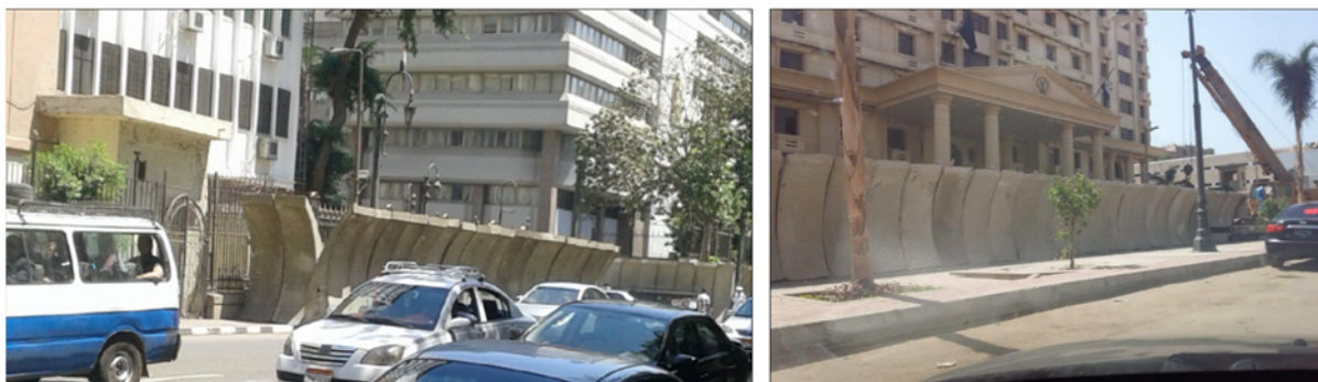
Figure 7. Left: Concrete blast shields installed next to the governmental buildings in downtown Cairo. Source: taken by the author in June 2015. Right: The blast shields are installed in other locations in Egypt in fear of possible terrorist attacks. Source: Masrawey.com
