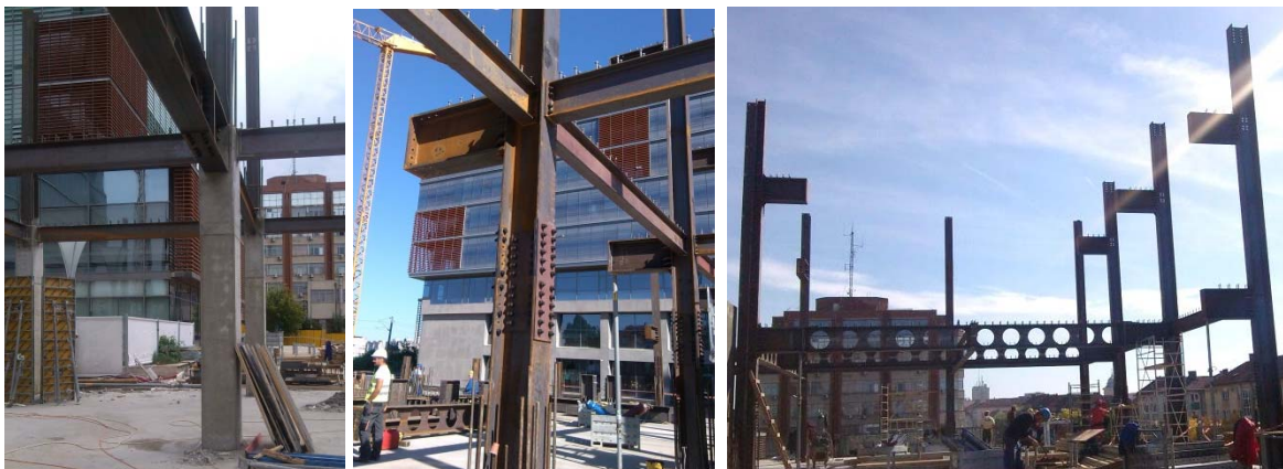
Figure 11. Composite columns during construction
