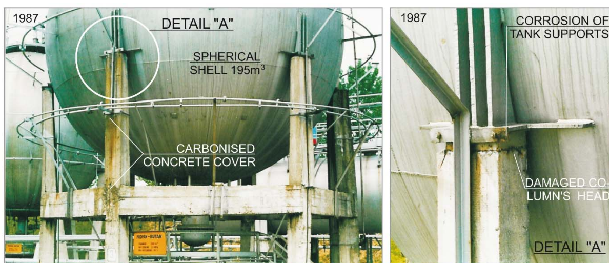
Figure 4. Structural faults of the support structures of tanks with a capacity of 195 m 3
