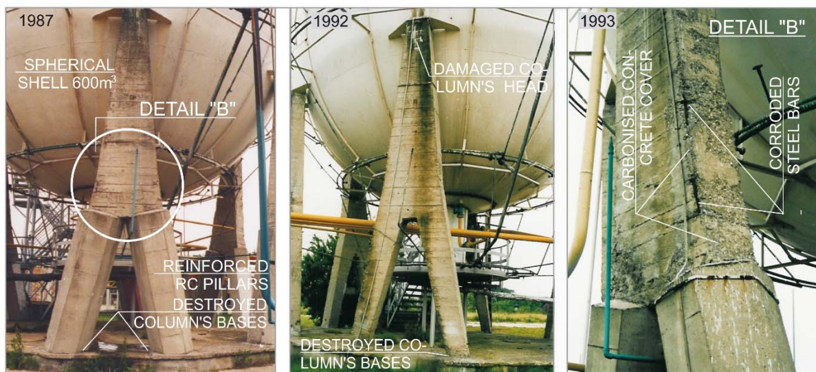
Figure 5. Structural faults of the support structures of tanks with a capacity of 600 m 3
