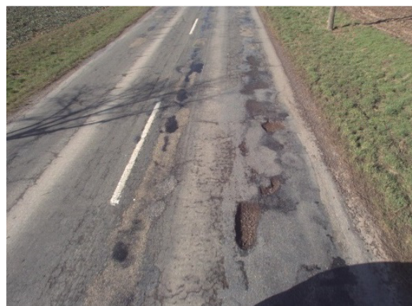
Figure 5. Digital photo of the same pothole on pavement.
