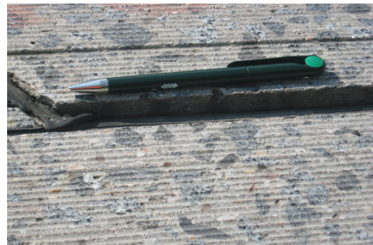
Figure 4. Detail of cracks in the left lane at the 76,000 km in summer 2010. grinded off.
