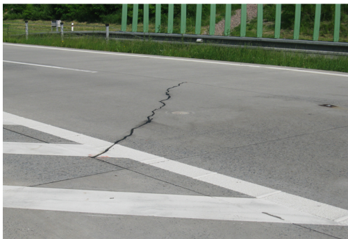
Figure 3. Disruption of the concrete road structure due to soil swelling, the direction of Prague.
