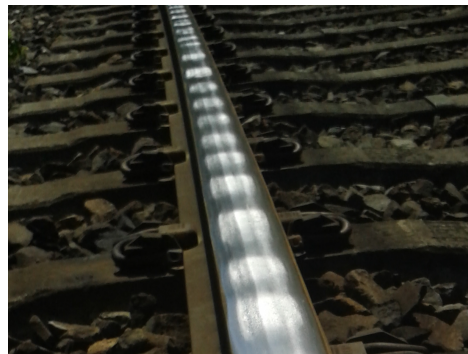
Figure 1. Long-pitch corrugation defect.
