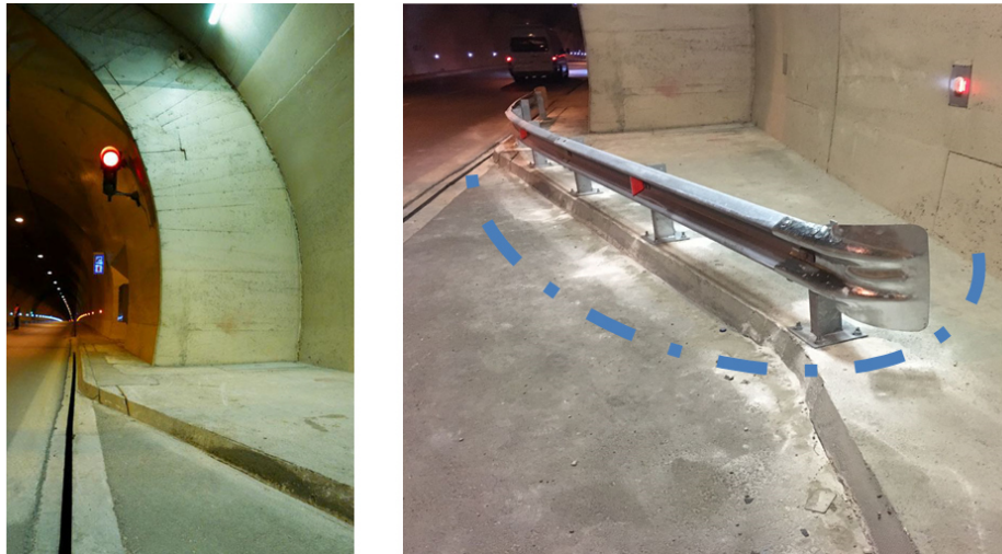
Figure 7. Installation of guardrail in front of perpendicular wall of lay-by in Krrabe tunnel (source: Hasani A., Albanian Roads Authority).
