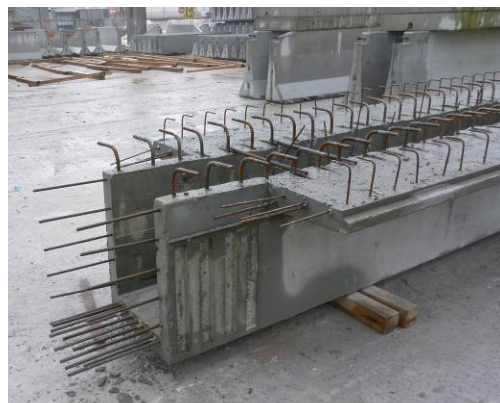
Figure 1. View of the end part of the Omega beam.
