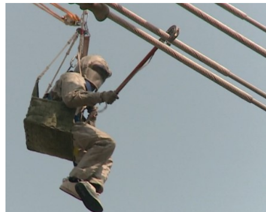
Figure 4. Field application of entering the electric field by the basket
