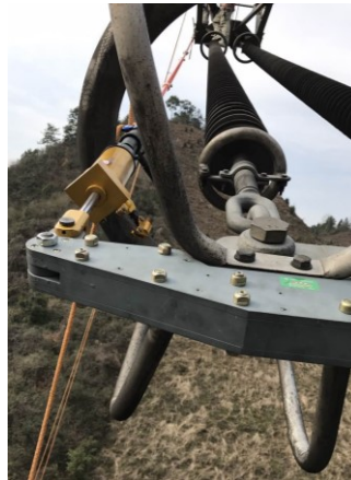
Figure 6. Field application of replacing the L-type insulator string by the new method
