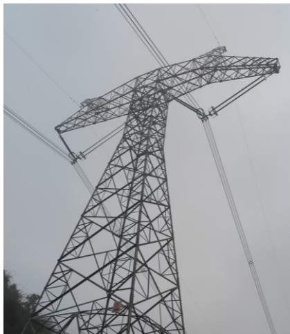
Figure 1. The field arrangement of L-type insulator string
