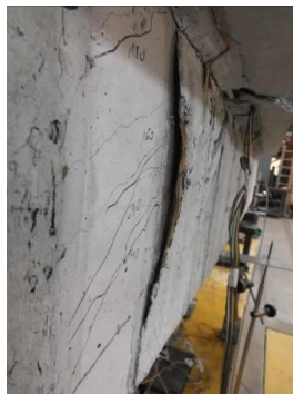
Figure 5. Failure of beam—debonding of the PBO mesh
