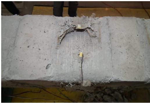
Figure 2. Failure of beam B1 – delamination of the lap on the top surface
