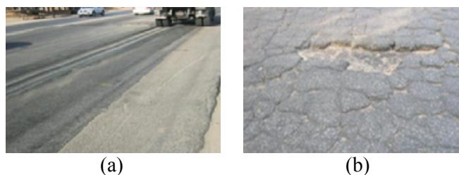
Figure 2. (a) Rutting; (b) Fatigue cracking
