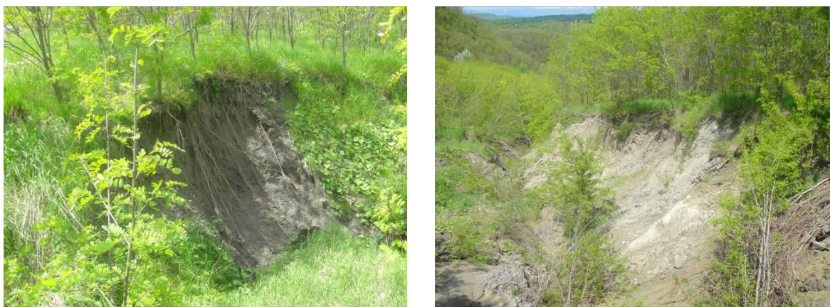
Figure 8. The case of Berbești tailing pond, Vâlcea county– instability phenomenon in area cultivated with acacia
