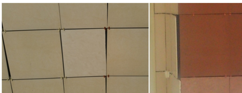
Figure 1. Defects of façade systems: facing walls design inconformity
