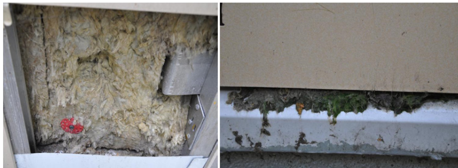
Figure 4. Result of hydro windproof membrane refusal
