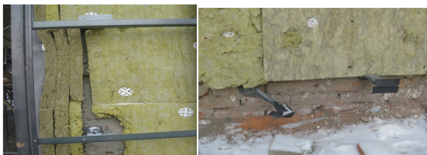
Figure 6. Defects in the process of overhead façade system installation
