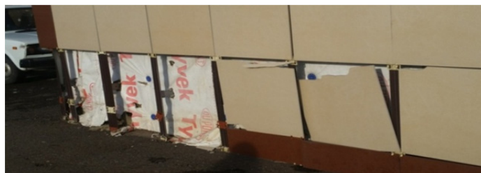
Figure 5. Destruction of the cladding material
