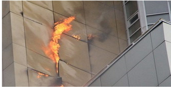
Figure 3. Membrane burning in the facade system design
