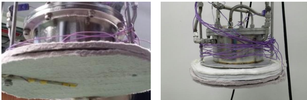
Figure 3. Basic installation of aerogel blankets under the cold mass tank and the heat absorber chamber; the bottom of the apparatus (left), the front of the apparatus (right)
