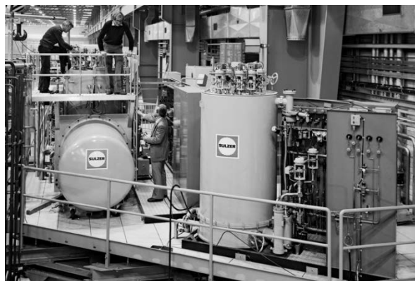
Figure 6. 400 W @ 4.5 K refrigerators (SULZER) in CERN North Area in the 1970s
