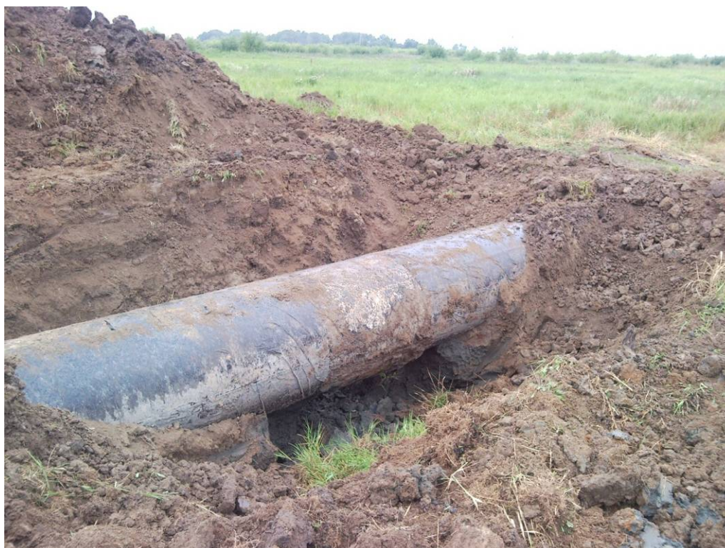
Figure 2. Check pit on the pipeline UBKUA made based on the results of the diagnostic test.
