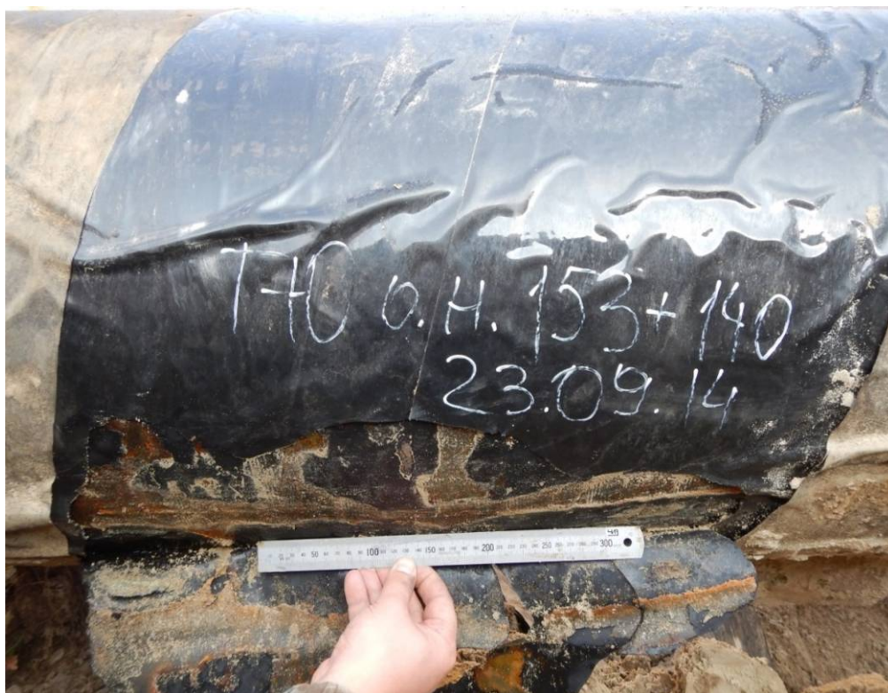
Figure 4. Check pit on the pipeline T-Yu made based on the results of the diagnostic test.
