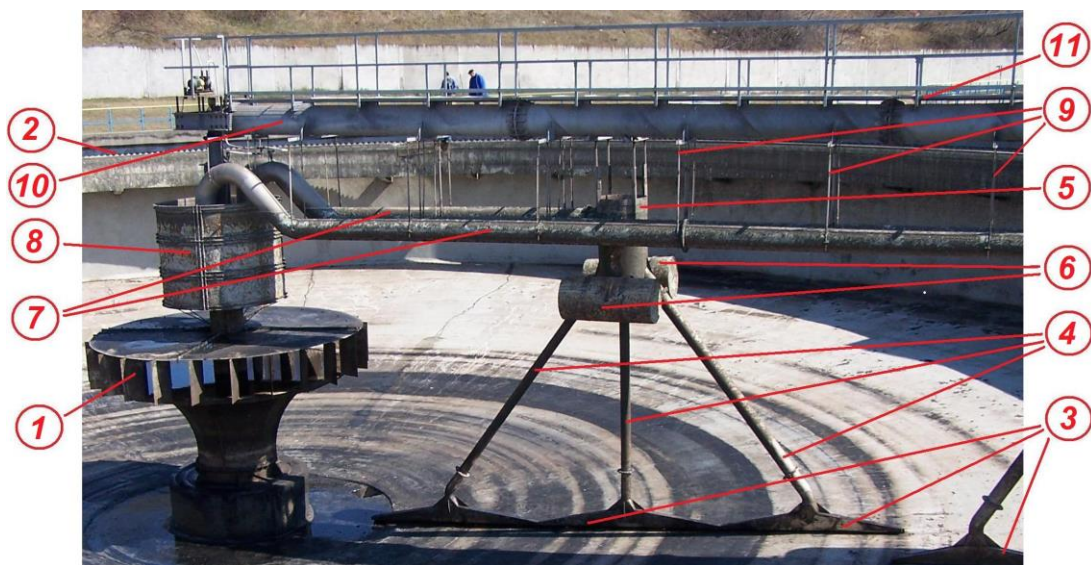
Figure 1. Components of the rotating half-bridge.
