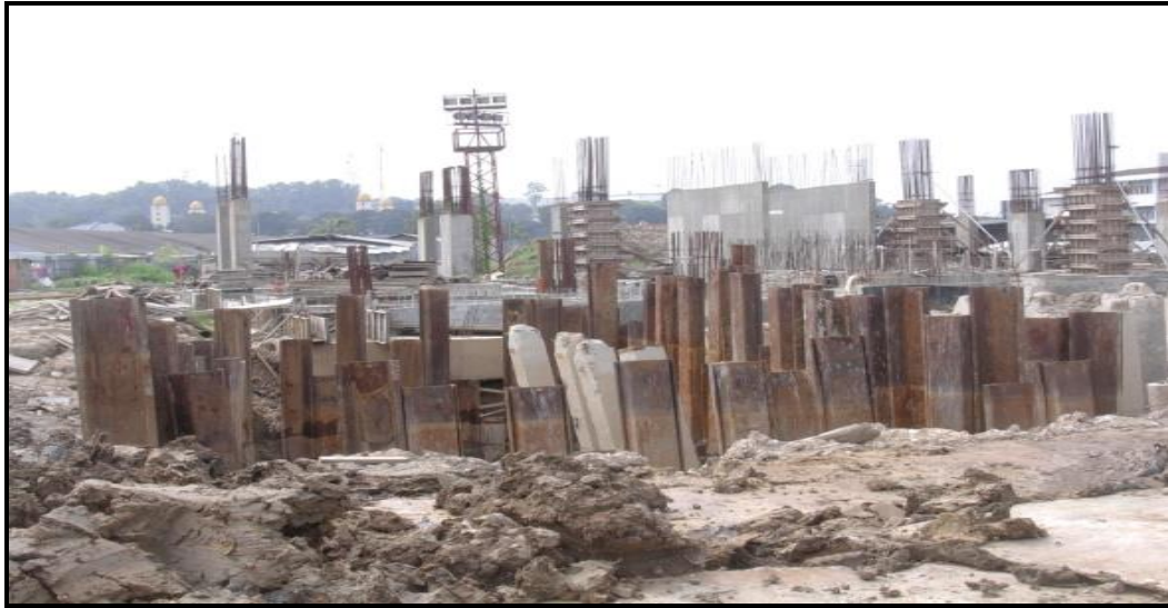
Figure 2. Sheet piles and piles adjacent to the excavation pit tilted.
