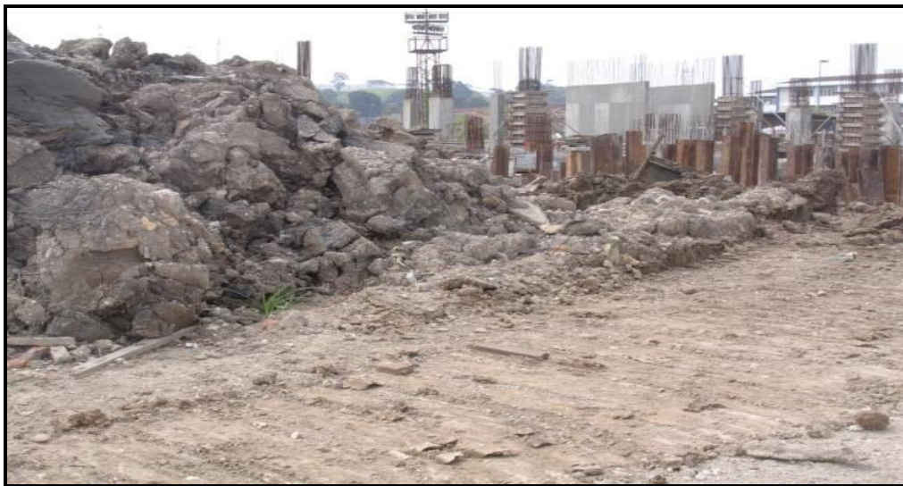
Figure 3. A large quantity of excavated earth dumped at the crest of excavation pit.
