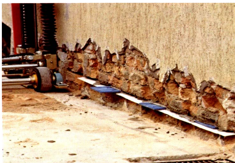
Figure 1. Introduction of anchoring wedges.
