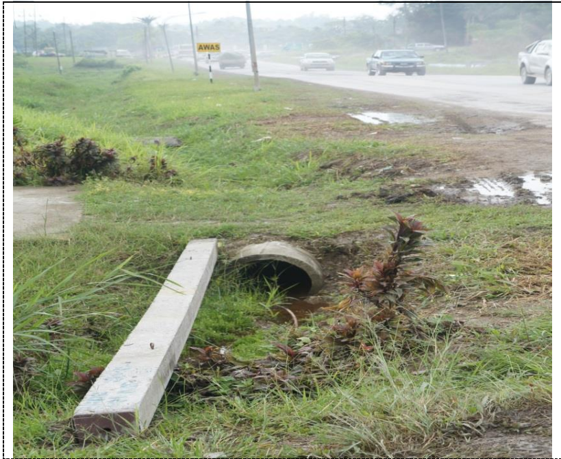
Figure 5. Blockage in part of a longitudinal drain in Road 2
