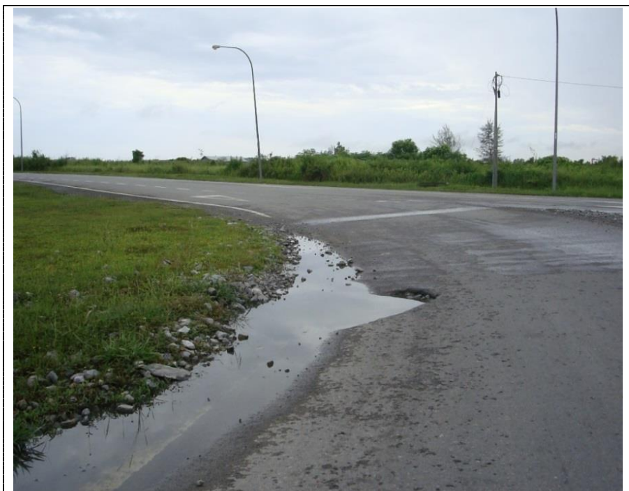
Figure 4. Accumulation of water on turning junction of Road 5
