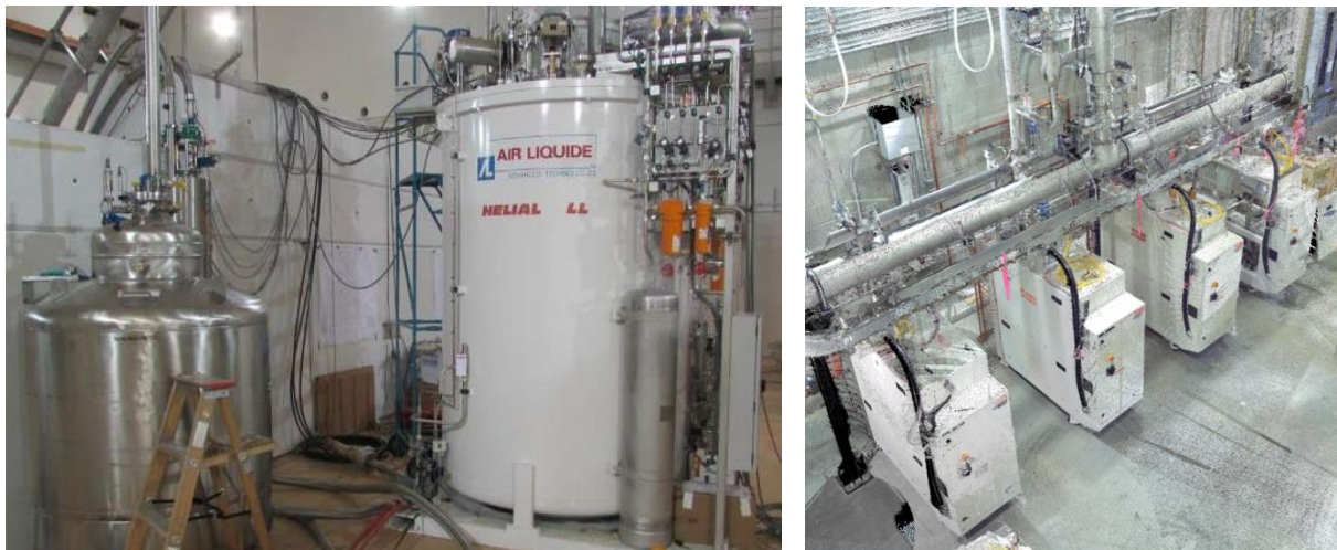
Figure 4. Helium cryoplant during commissioning phase (a); S/A pumping system (b)
