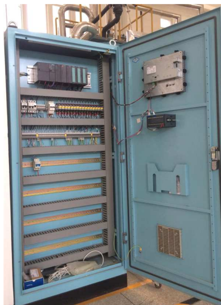
Figure 2. The I/O Module cabinet of 10kW@20K large scale helium refrigerator.
